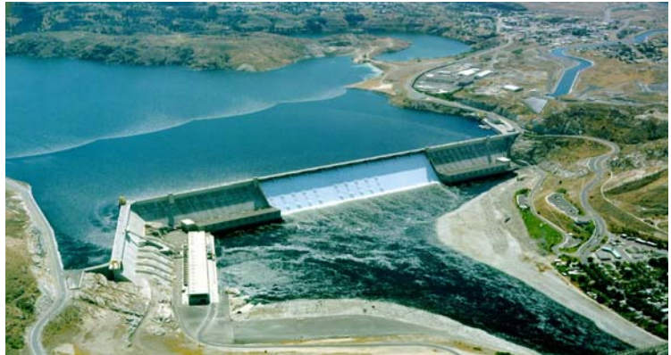
The massive Grand Coulee dam, whose controllable reservoir capability contributes to the uncertainty in regional hydro generation, can generate nearly 6,500 MW of power.
